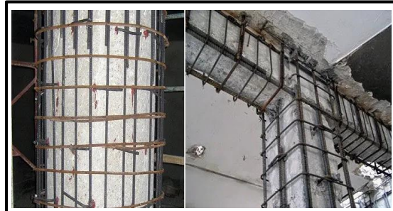
Fig. 14.10 Column Beam Jacketing
