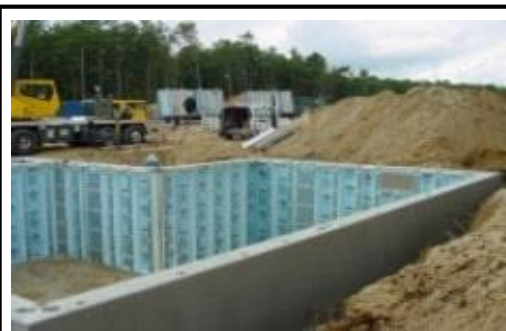
Fig. 14.15 Precast Concrete Foundations
