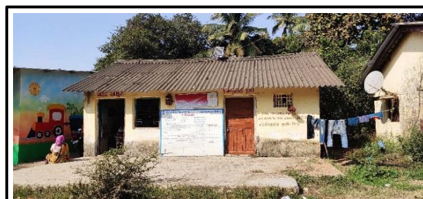
Fig 4.27 Post Office and Community Hall
