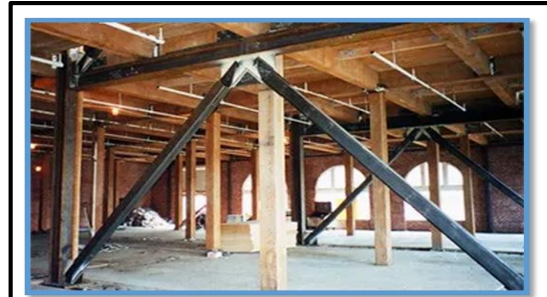
Fig. 14.6 adding steel bracing
