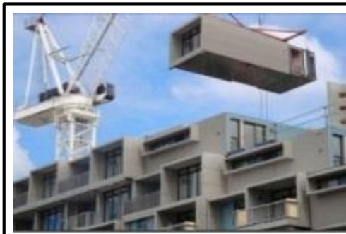
Fig. 14.13 3D Volumetric Construction
