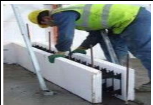
Fig. 14.17 Insulating Concrete Formwork
