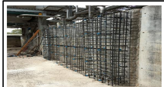
Fig. 14.7 Wall thickening technique
