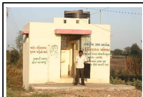
Fig 1.18 Baben Village Public Toilets
