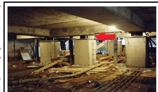
Fig. 14.8 Base isolation technique
