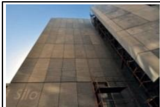
Fig. 14.18 Precast Cladding Panels
